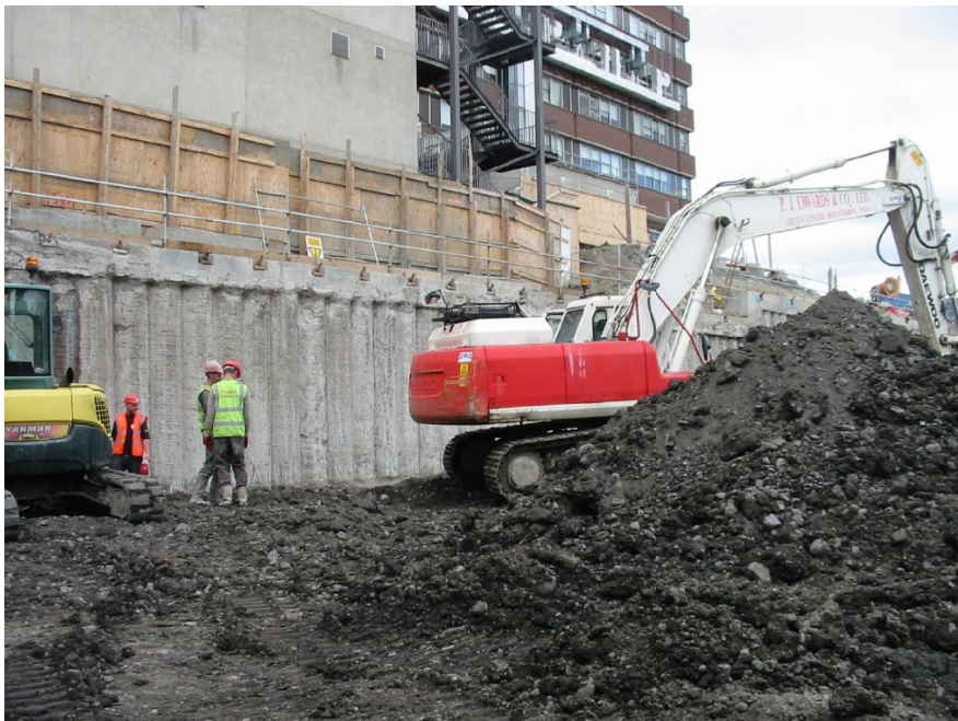
Figure 13 : Secant Pile Works in close proximity to Existing Buildings
